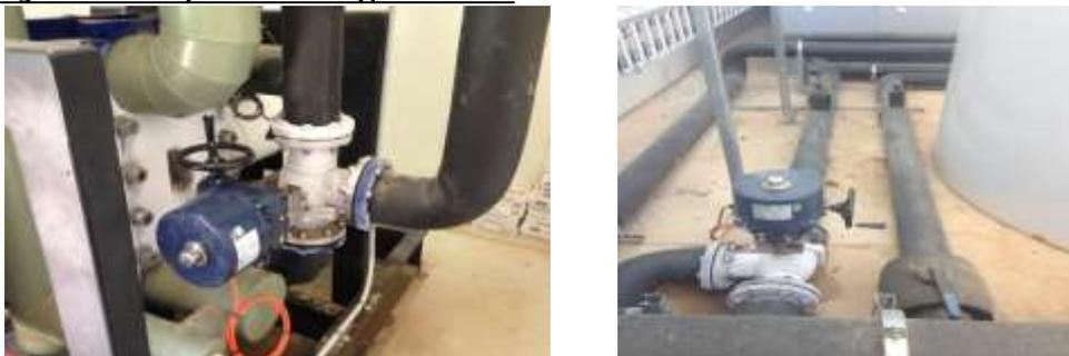
Figure 13 shows the Dynalene circulating and process pumps. Each room has its own Dynalene process pump,  $-6^{\circ}\text{C}$  Dynalene is pumped to each of the room evaporators, from there it returns back to the warm Dynalene tank.
